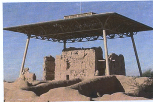
Figure 1. Casa Grande Ruins National Monument structure composed of earth, which is covered by a roof to protect it from erosion. In the foreground are walls that have been preserved with modern coating material to protect them from natural erosion.
