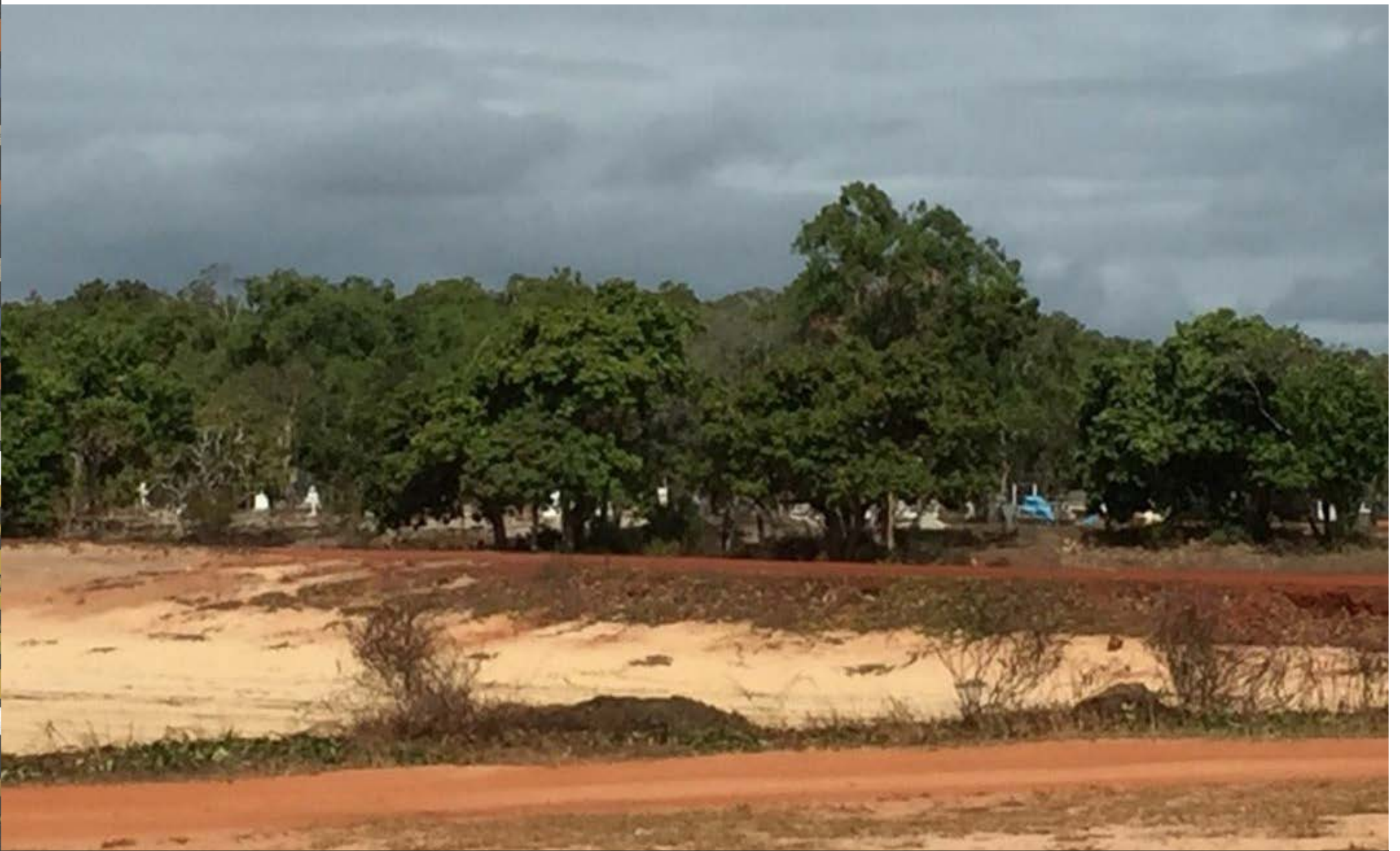
Overview of Injinoo Cemetery, Queensland, showing the threat of coastal erosion to the cemetery boundary. A threat that is expected to increase over this century with ongoing climate change and sea level rise.
